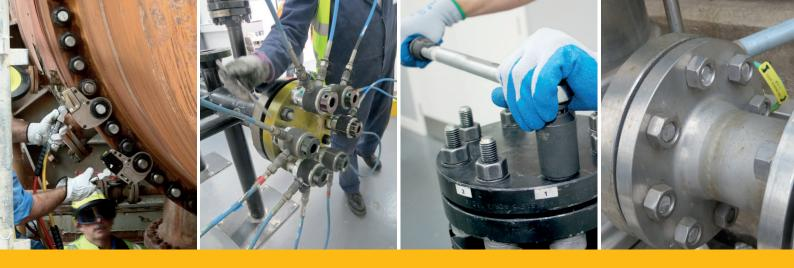
**To ensure** the optimum level of resources and verification is carried out on each joint, a criticality assessment will be carried out, which will consider the service, pressure and local <u>conditions of each connection</u>.
